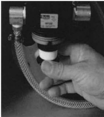
4. Separate the filter from the filter holders. Replace with a new filter.
